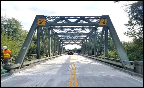
Samish River Bridge - Vertical Clearance Signage
