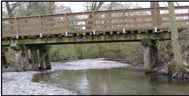
Cascade Trail Bridge at Jones Creek
