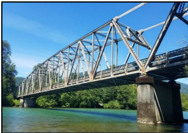
Marblemount Bridge – Skagit River
