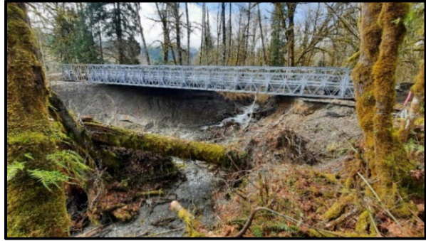
Temporary Bridge over North Osterman Creek, looking upstream.
