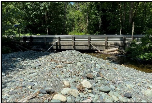
Mill Creek channel upstream of bridge.
