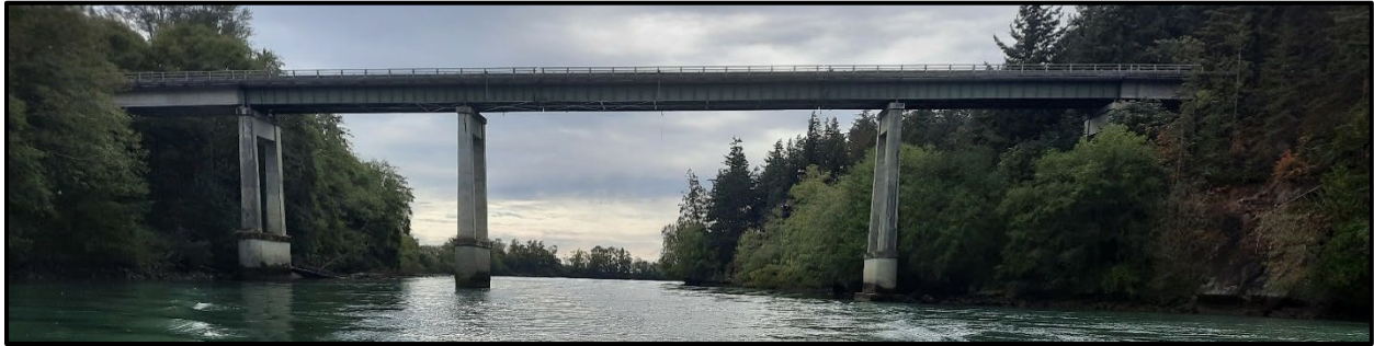
North Fork Bridge looking downstream.
