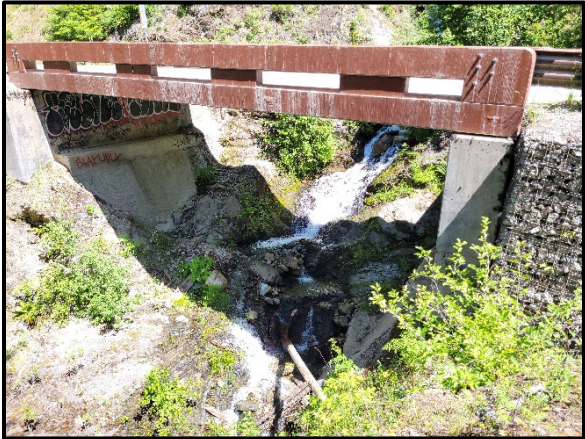
Cascade River Road at Hard Creek Bridge, looking north, upstream.
