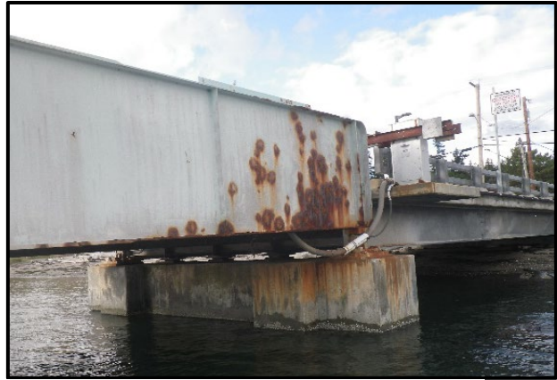
M/V Guemes Ferry Anacortes Terminal – Transfer Span
