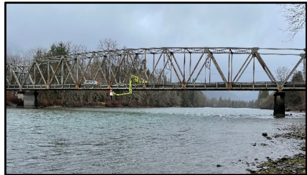
Skagit River Marblemount Bridge, UBIT inspection
